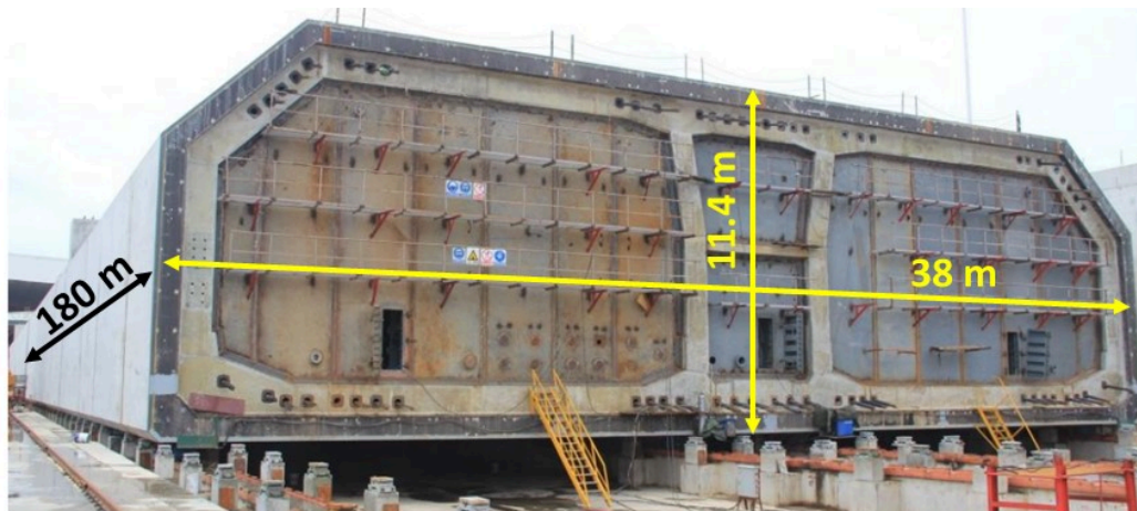
Fig. 1 – View and dimensions of tunnel precast segments of Hong Kong – Zhuhai – Macao link
